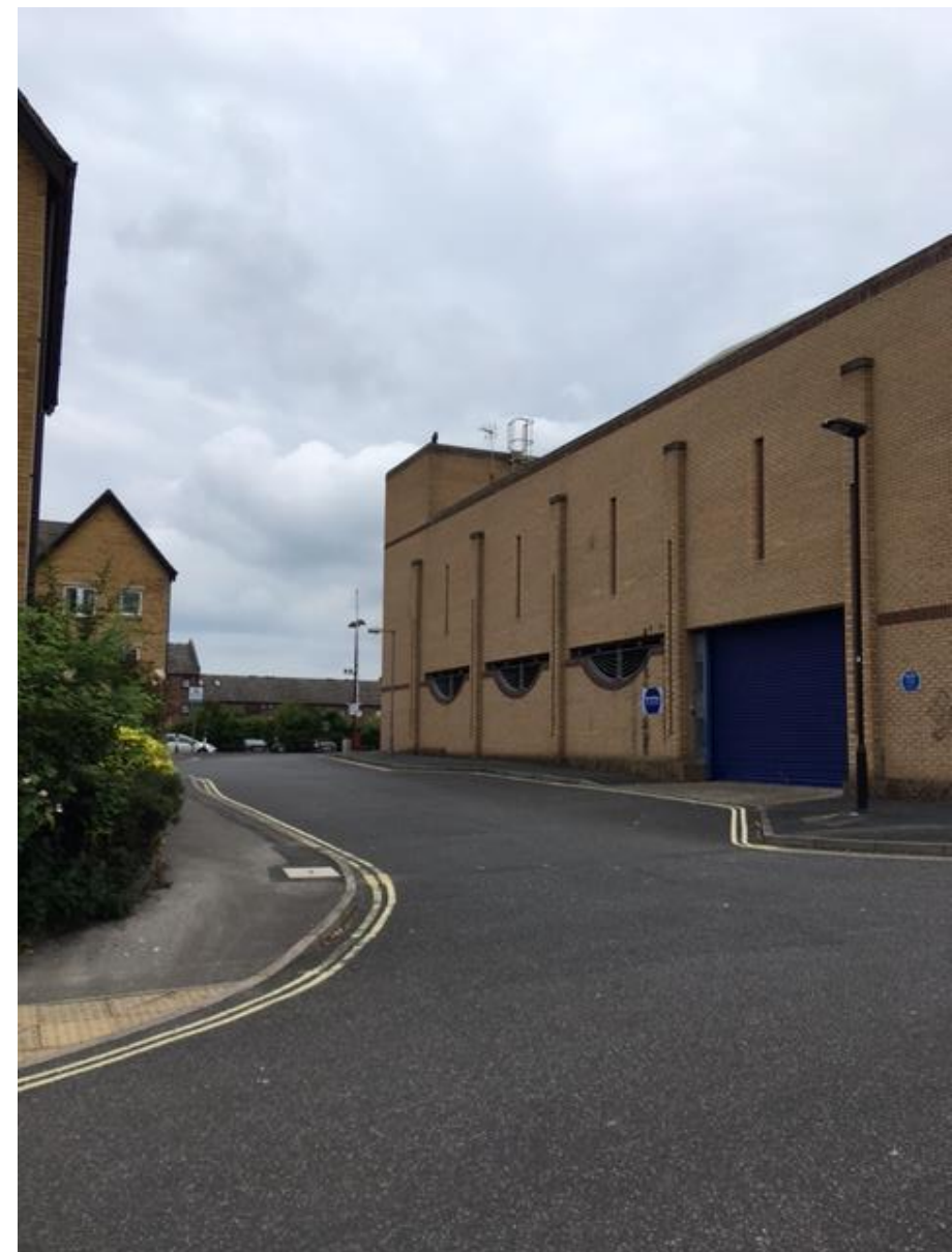
Rear Elevation Facing South/William Court
